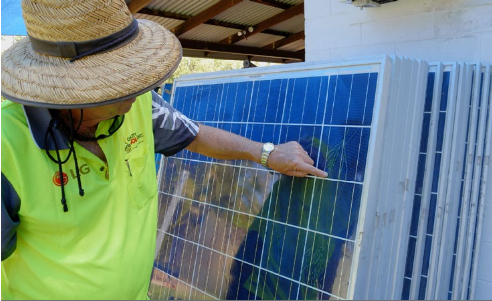
Inspecting cheap panels, that failed after 3 years and were pulled off the roof. The consumer was unable to claim against the manufacturer who had left Australia.
